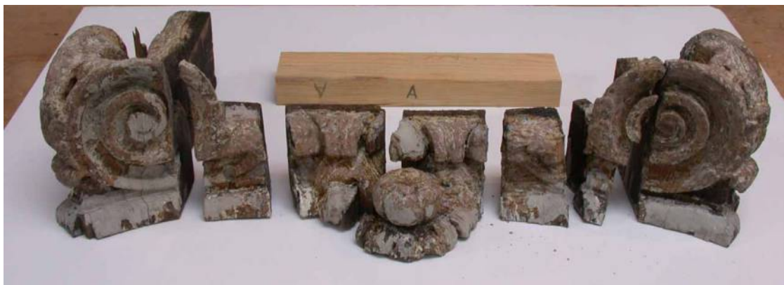
FIG. 1. One of four capitals from Mount Pleasant, shown inverted and in fragments after removal of roughly 20 layers of paint. Attributed to Bernard and Jugiez, Philadelphia, 1762–1765, southern yellow pine, 9.8 \times 29.8 \times 15.7 cm ( H \times W \times D ), Philadelphia Museum of Art.
